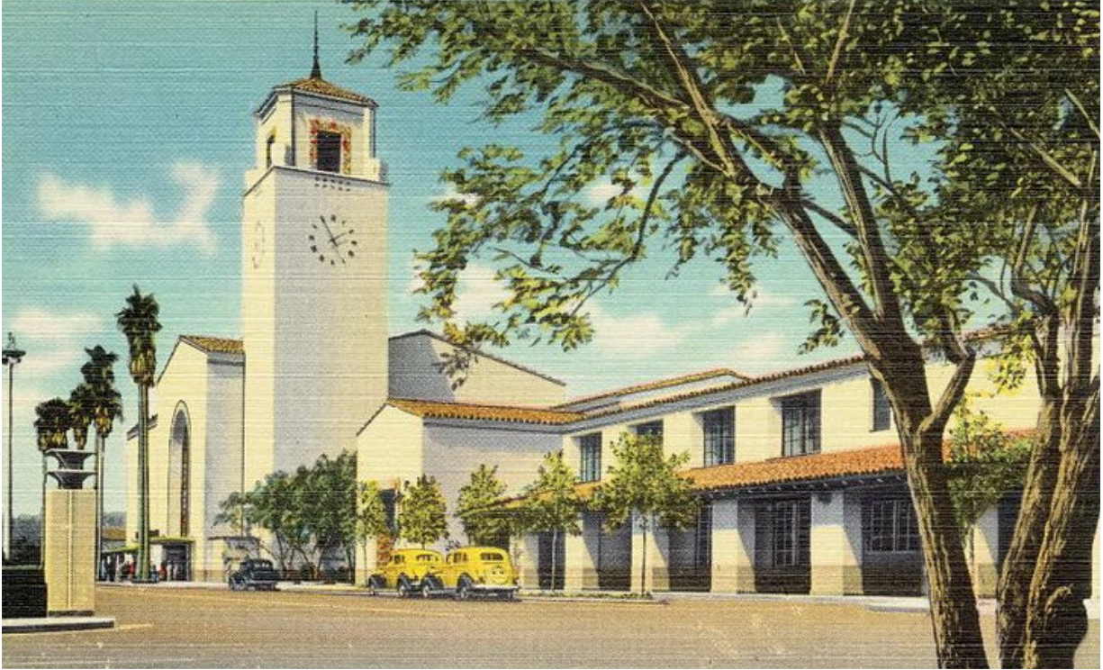
Figure 14.1: Union Station of Los Angeles, The Largest Passenger Terminal in the Western U.S. (Circa 1930) 164
