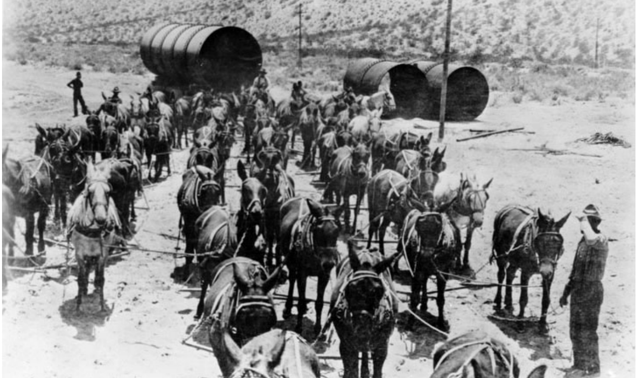
Figure 5.1: Borax Mules Pulling Aqueduct Pipes for Installation in the Owens Valley. 43
