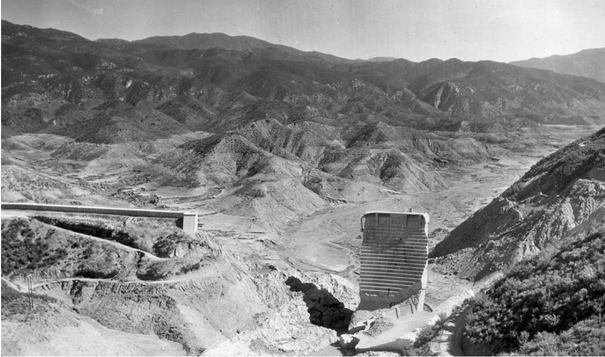
Figure 5.9: The Aftermath of the St. Francis Dam Collapse, 1928. 53
