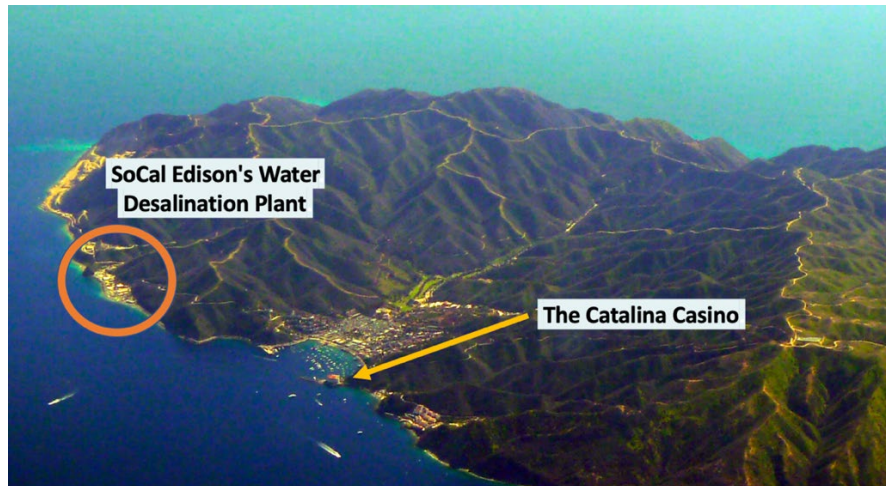
Figure 5.5: Catalina Islands Desalinization Plant. Image Source: 49
